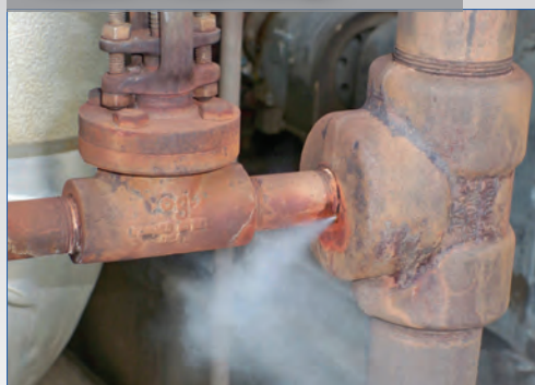
FIGURE 7: Steam leakage.
