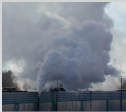
FIGURE 1: Significant steam losses = significant dollar losses. All images courtesy: Inveno Engineering/ESC
